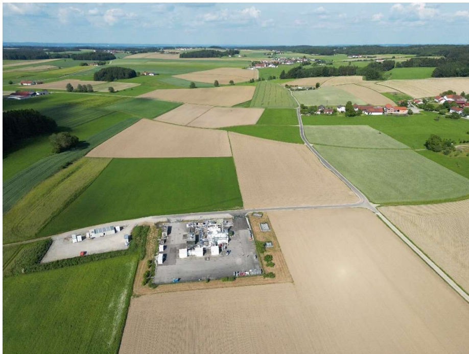
Looking at the BW B6 drilling site at the Bierwang storage site. The HyStorage research project is carried out here. (Source: Uniper Energy Storage)
