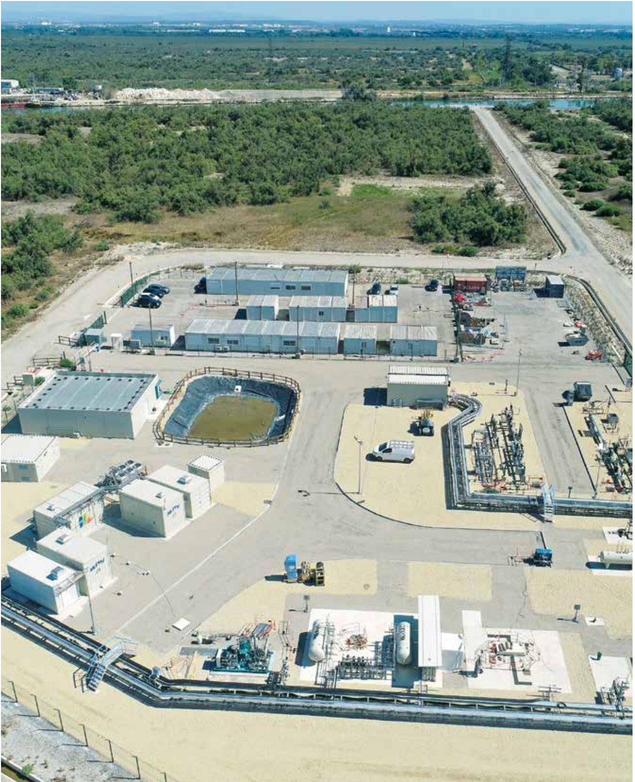
↑ The Jupiter 1000 project, coordinated by GRTgaz, is the first industrial demonstrator of Power to Gas in France with a power rating of 1 MWe, converting renewable power surplus into green hydrogen and syngas for storage.
